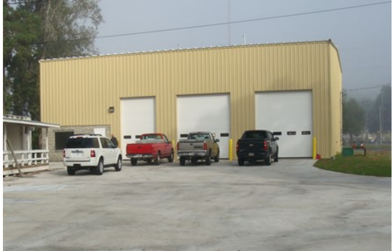
Glynn County Fire Department maintenance building
