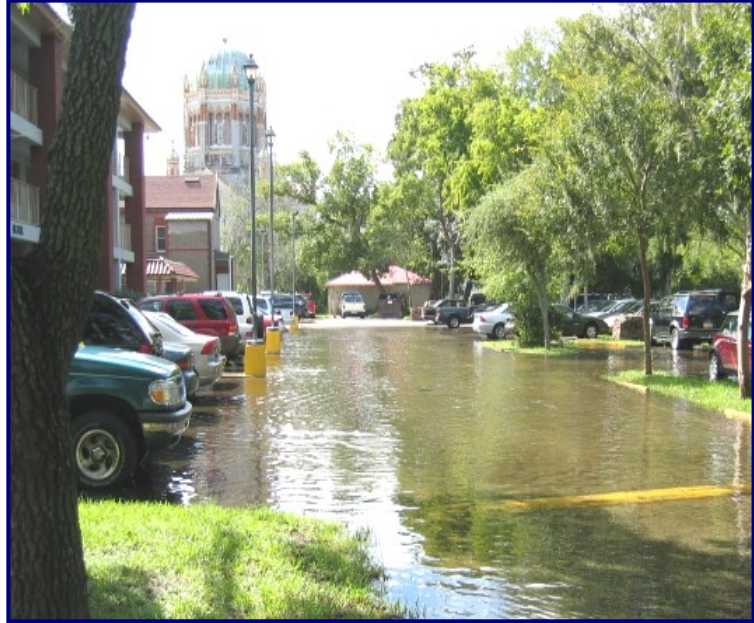
Flooding in Lewis Hall parking area
