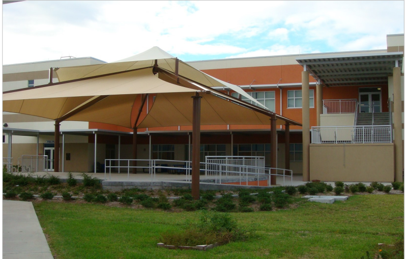
The two-story, 16-classroom addition to the school complex opened for the 2011 – 2012 school year.
